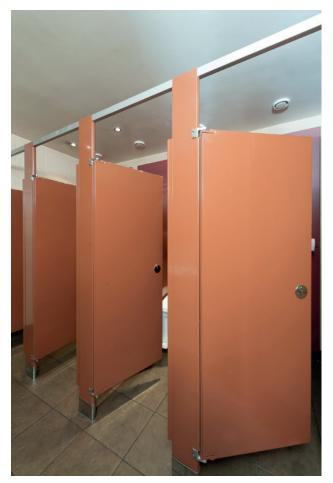
What they needed were cubicles that were much more durable, would look good for years and could harmonise with the shade of purple/brown that featured elsewhere in the room. Hadrian Elite steel cubicles from Relcross were chosen and specified in RAL 8002 Signal Brown. These floor mounted, overhead braced toilet partitions are especially suitable for heavy use areas and require no special structural provisions to effect a rigid installation. They can be erected on any type of floor.
