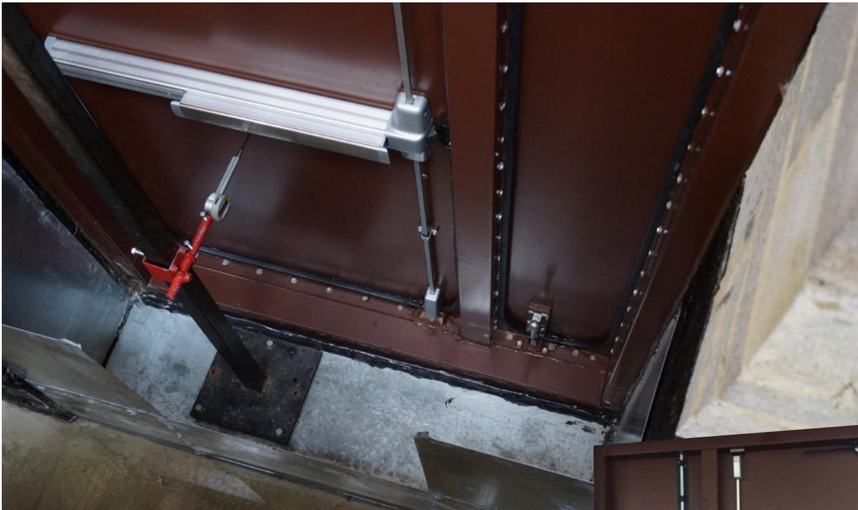
Slight pressure anywhere on the pad simultaneously retracts all 3 latches at the top, bottom and side of the door allowing it to open quickly and reliably time after time. In fact Von Duprin 99 escape devices have been independently tested to 5 million cycles and are also CE marked for complete peace of mind. As well as their durability they are also renowned for their integral fluid dampener that reduces noise and creates a smooth and almost silent operation.
