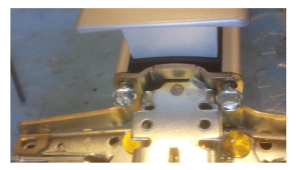
Remove these and any screws fixing the latch and body to the door and remove the clip to allow the back-plate to be removed from the aluminium extruded body.
